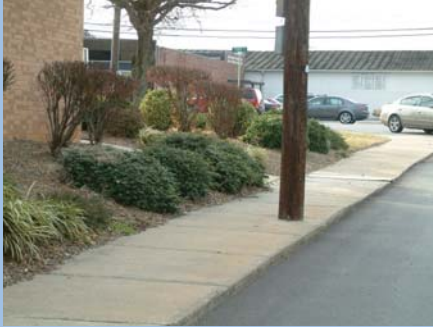
Specific segments of sidewalk in downtown Yadkinville lack sufficient width for ADA access
