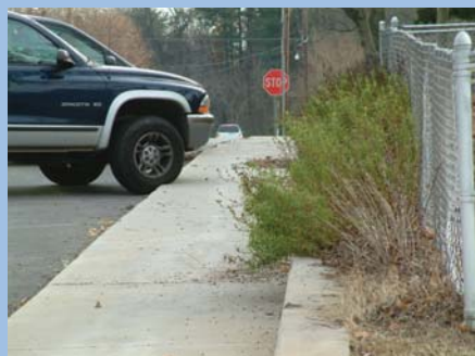
Installing curb-stops will prevent cars from potentially jumping the curb and will keep pedestrians safe
