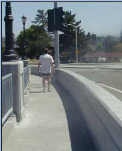
Pedestrian sidewalk on bridge with separation. Photo credit: www.fhwa.dot.gov
