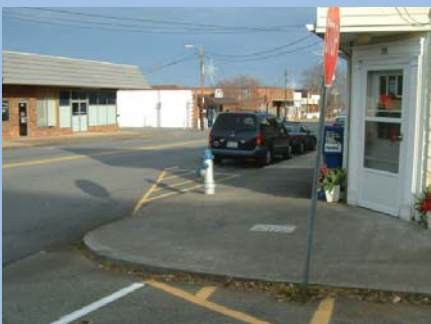
Non-compliant ADA Curb and Gutter
