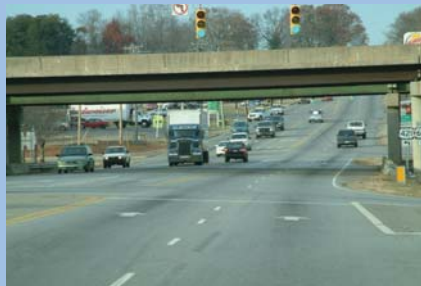
US 421 Hwy Bridge underpass
