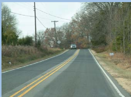
Narrow road shoulders make walking between destination dangerous on US 601 Hwy South.
