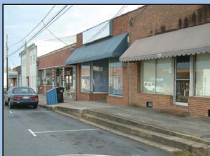
Grade changes on portions of Main Street make sidewalk ADA access difficult
