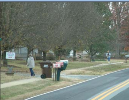
Even with proper separation from vehicles, sidewalks need to be free of obstructions for ADA accessibility
