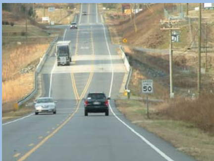
View looking of US 601 Hwy South towards southern Town Limit
