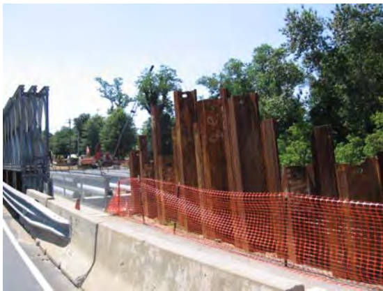
Bridge Replacement on Main Street Above the Deep River
