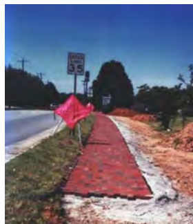
Sidewalk Installation Main Street
