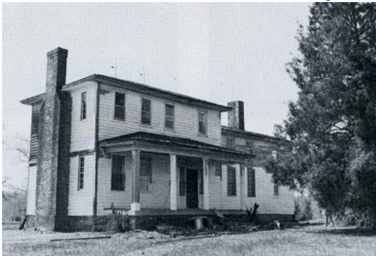
Jeduthan Harper House, ca. 1800 Courtesy Architectural History of Randolph County, NC
