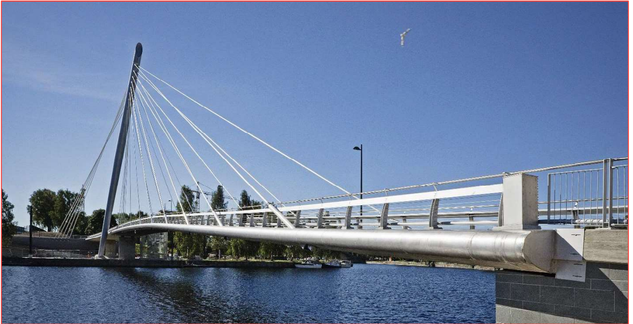
Figure xi: Laukonsilta Pedestrian Bridge
