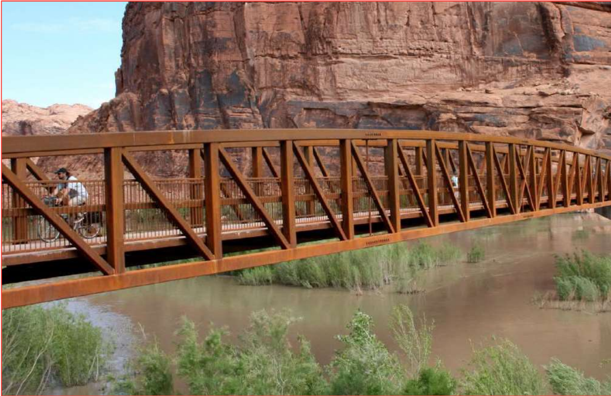
Figure vii: Colorado Riverway Bridge (Capstone Truss Style, Weathering Steel).
