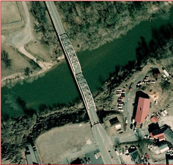
Figure i: Hugh Chatham Memorial Bridge (2007)
