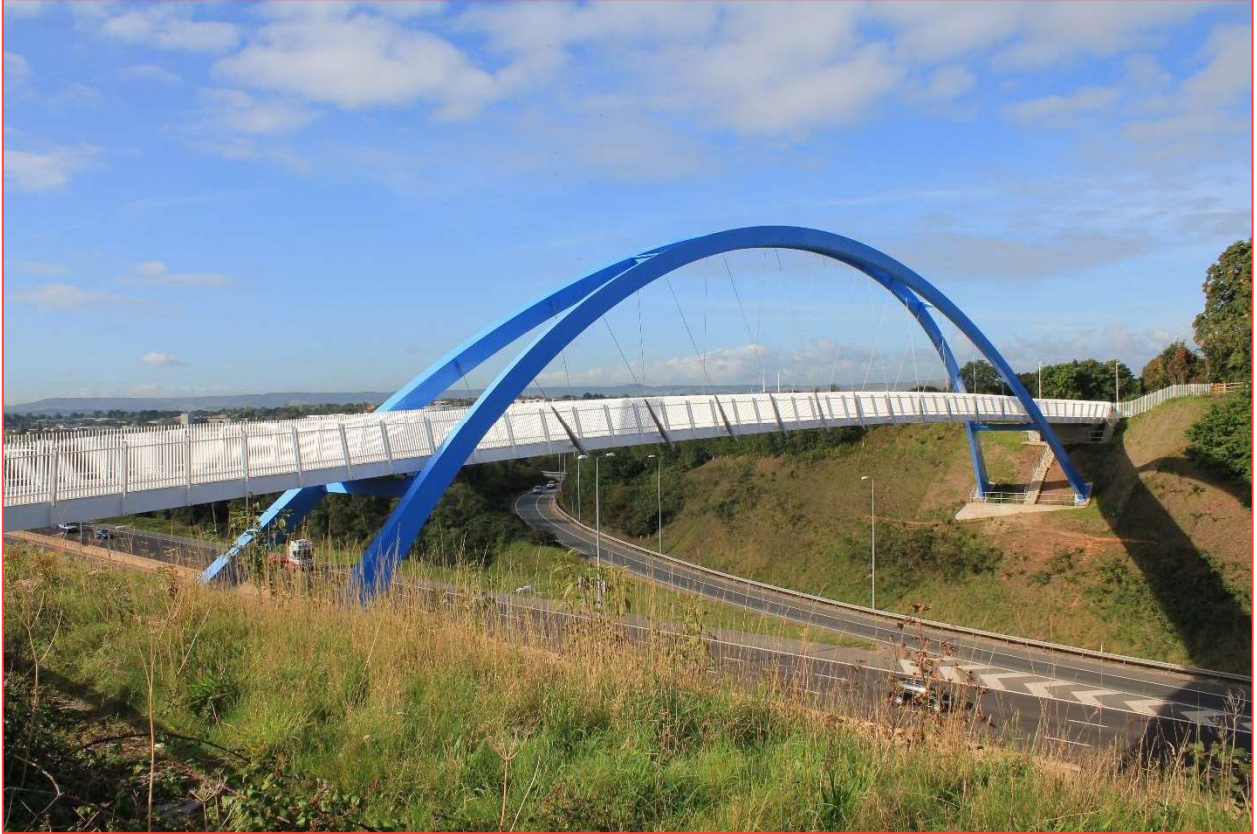
Figure x: Redhayes Bridge M5
