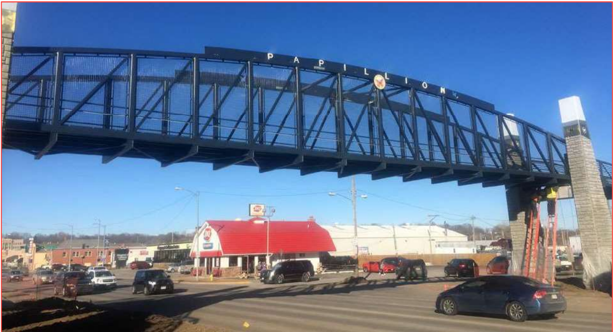
Figure viii: 84 th Street Crossing (Capstone Truss Style, Painted Steel).
