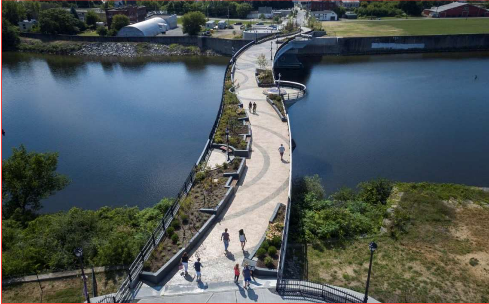
Figure xvi: Mohawk Valley Gateway Overlook Pedestrian Bridge
