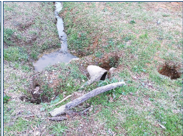
(Left) Safety issue - broken asphalt with unsecured grate placed on top (Right) Exposed pipes and sinkholes, evidence of surface and overland flow
