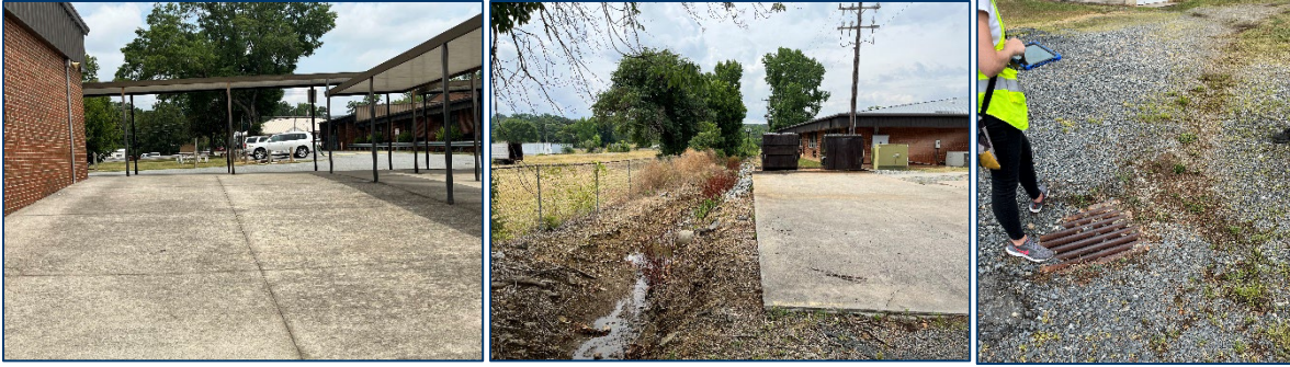
School grounds contain lots of impervious surfaces, unvegetated drainage ditches, and unmanaged drainage areas
