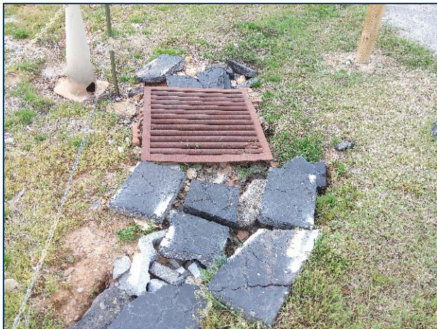
(Left) Safety issue - broken asphalt with unsecured grate placed on top (Right) Exposed pipes and sinkholes, evidence of surface and overland flow
