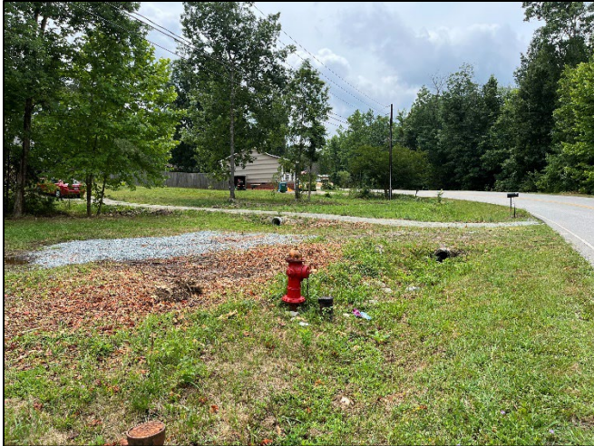
Clark Acres at Old Camp Road: Road is pitched; three different inlet pipes lead to three open channelized areas, draining to Old Camp Road; Map image on right shows elevation change to the corner of Old Camp Road.
