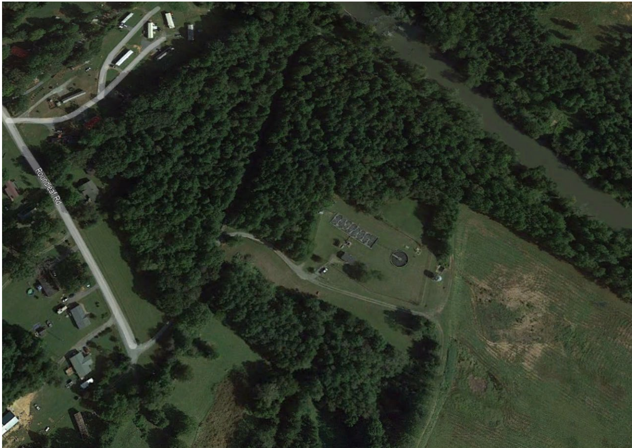
Image 2: The Ramseur wastewater treatment plant
