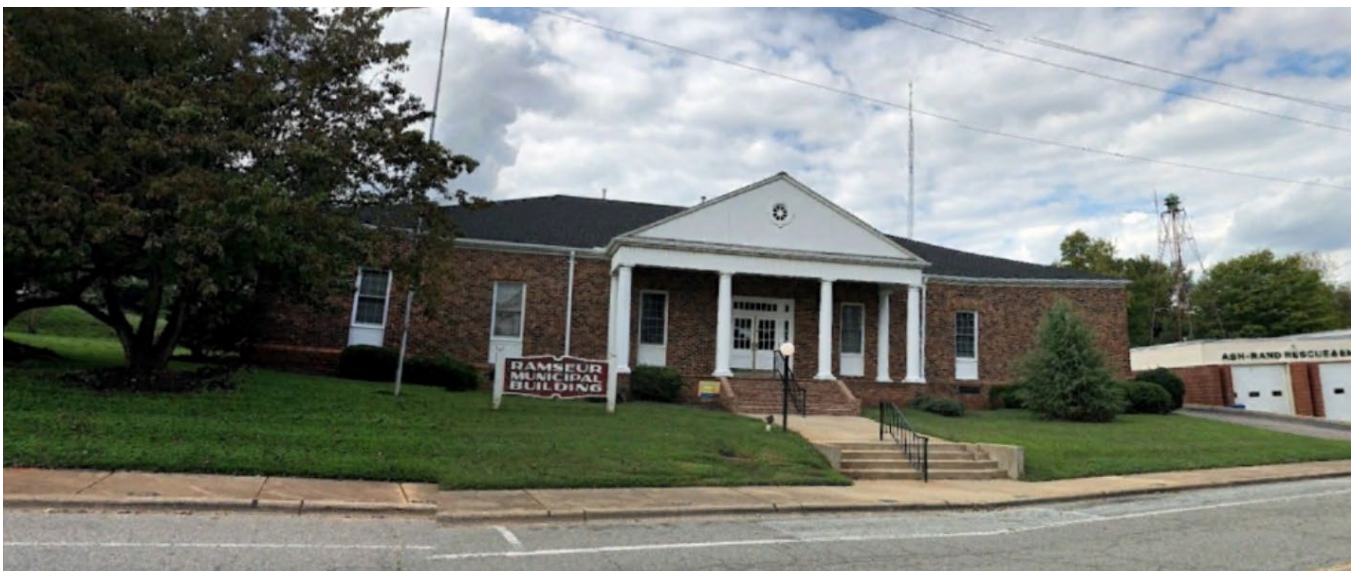
Ramseur Municipal Building
