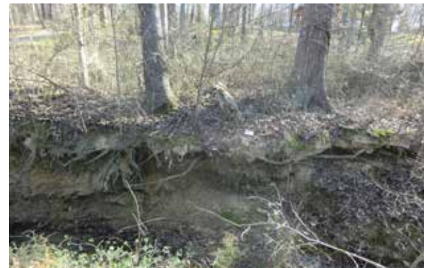
Figure 21: Improve major erosion along stream bank
