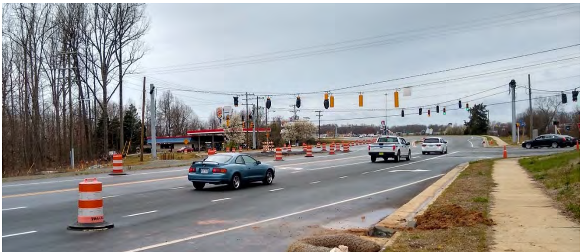
Figure 57: Roadway Improvements under Construction in Mebane
