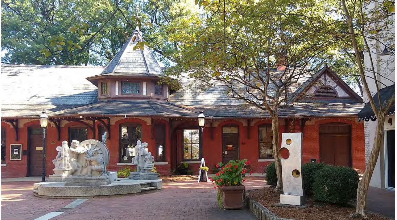
Figure 13: Southern Railway Passenger Station in Downtown Burlington
