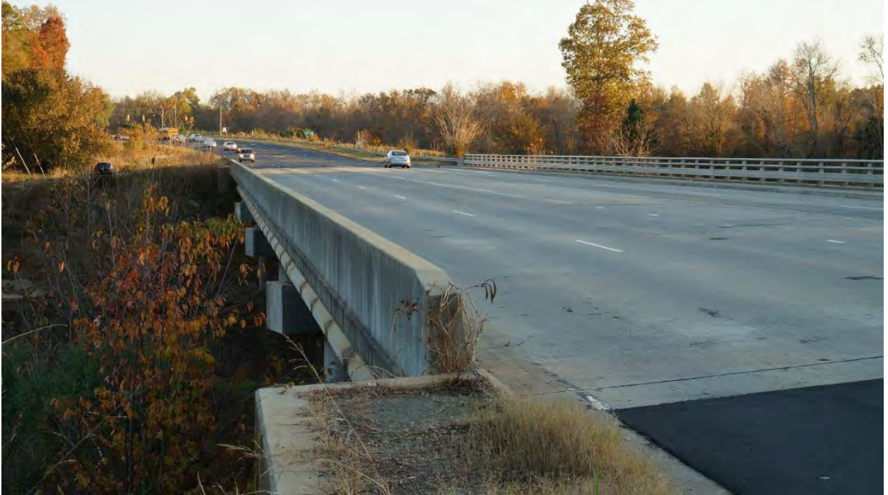
Figure 22: NC 54 Bridge over the Haw River
