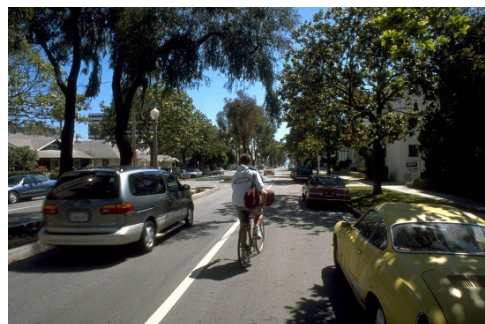
Example of an avenue with bike lane, on-street parking and a median.
