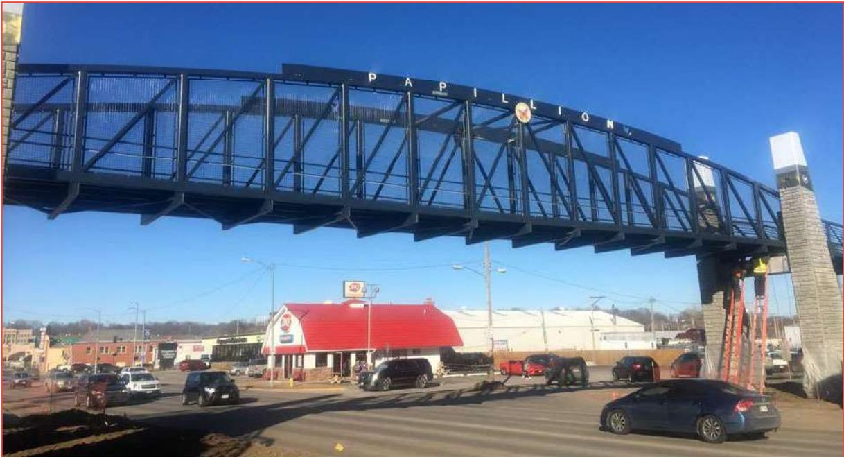
**Figure viii: 84<sup>th</sup> Street Crossing (Capstone Truss Style, Painted Steel).**
