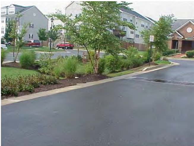
Figure 69: Rain Garden Collects Roadway Runoff (Source: LID Center)
