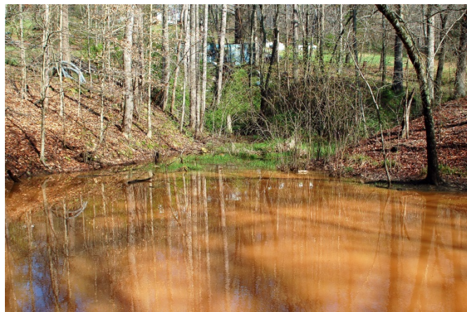
Figure 27: Failing Farm Pond & Spillway, Matrimony Creek, PTRC 2012
