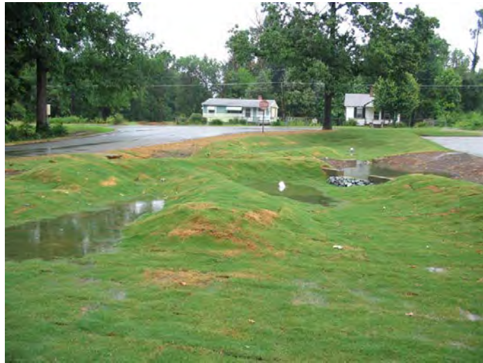
Figure 40: Alamance High School Bioretention Cell - Graham, NC
