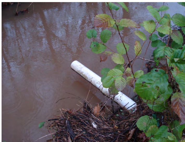
Figure 41: Illicit Discharge to Abbotts Creek
