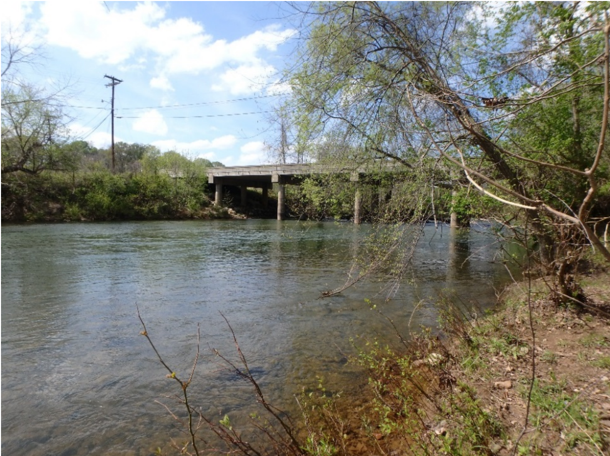
NC 135 Bridge on the Mayo River
