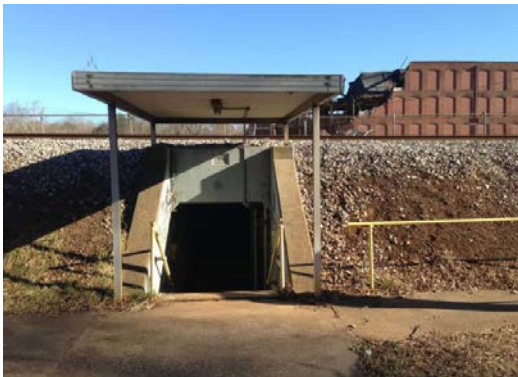
Tunnel From Recreation Center Property to Washington Mills Site
