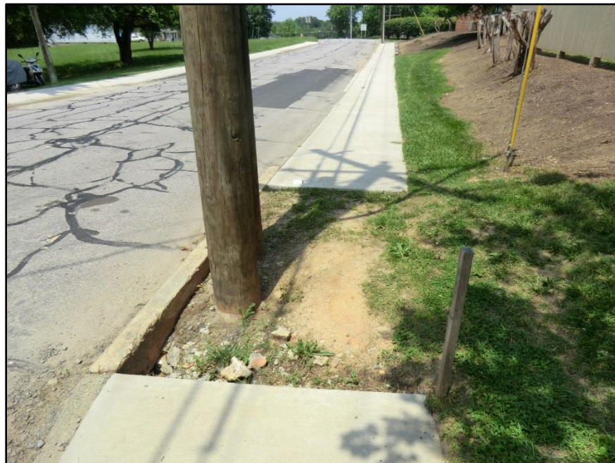
Figure 3: Sidewalk Gap Looking North Inside Study Area
