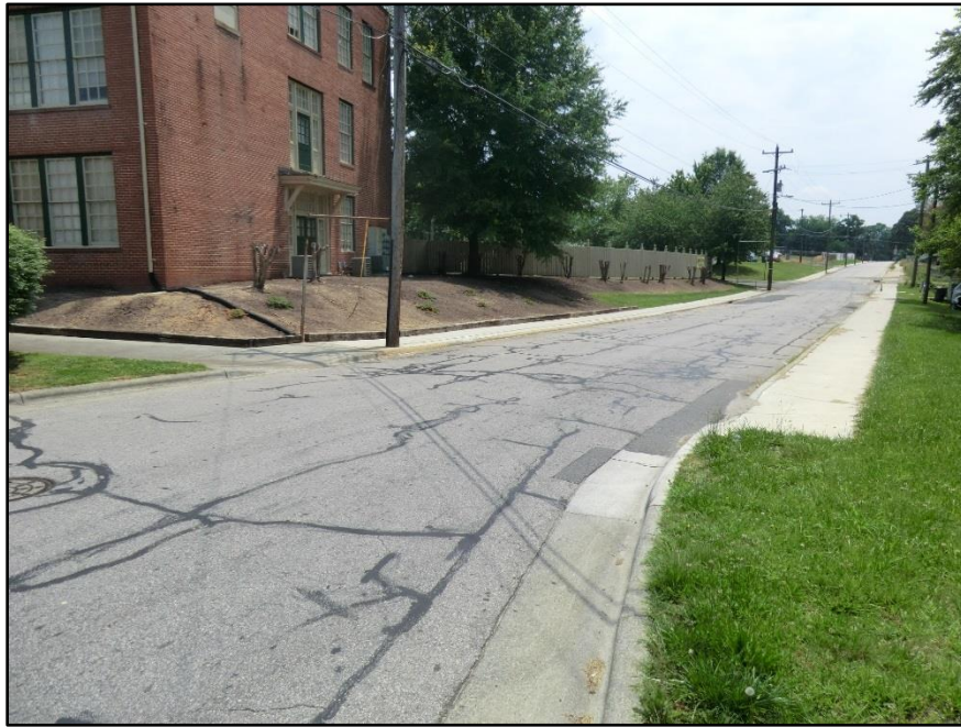
Figure 2: Location of Sidewalks Looking South Inside Study Area
