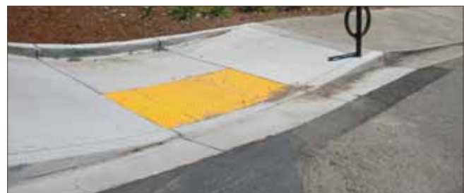
ADA compliant curb ramps
