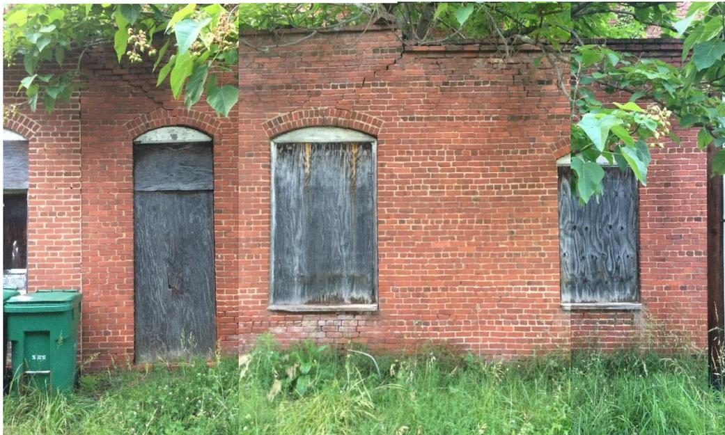
*Composite photo showing cracked brick walls requiring steel plate stabilizers.*
