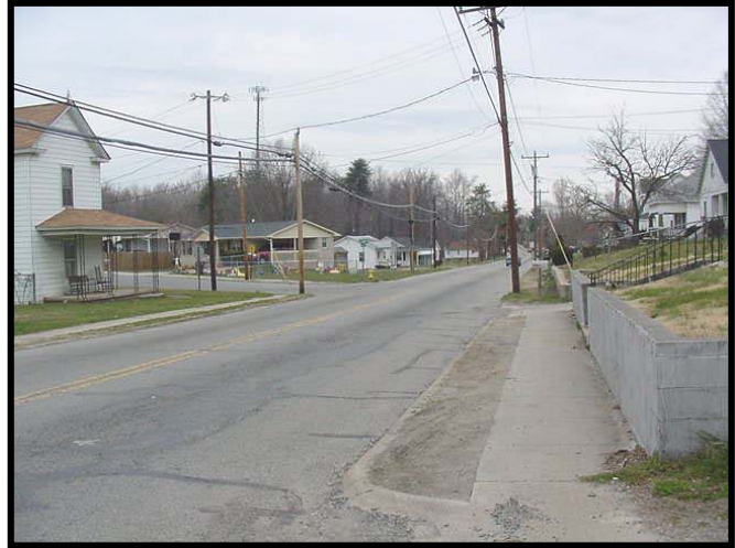
The existing North Scales Street corridor.
