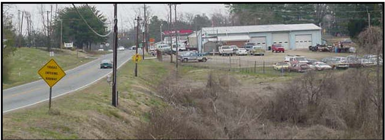
There are multiple opportunities for improving Reidsville's community image along its key entranceways.
