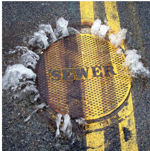
Figure 30: Sewer Overflow
