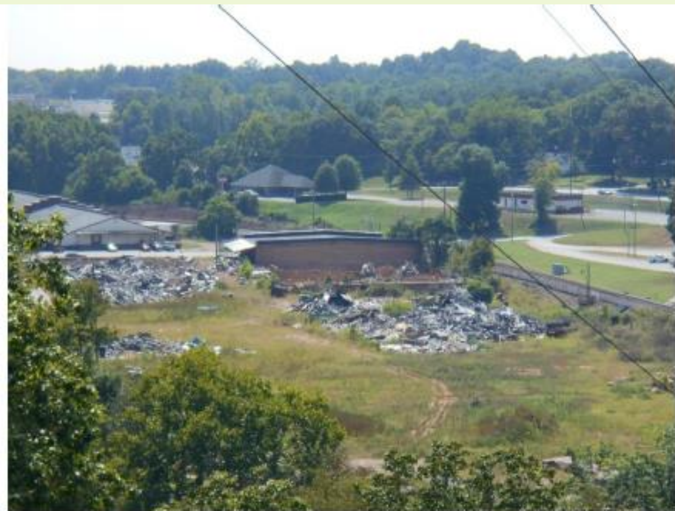
Photograph 1: General overview of the Site, looking south.
