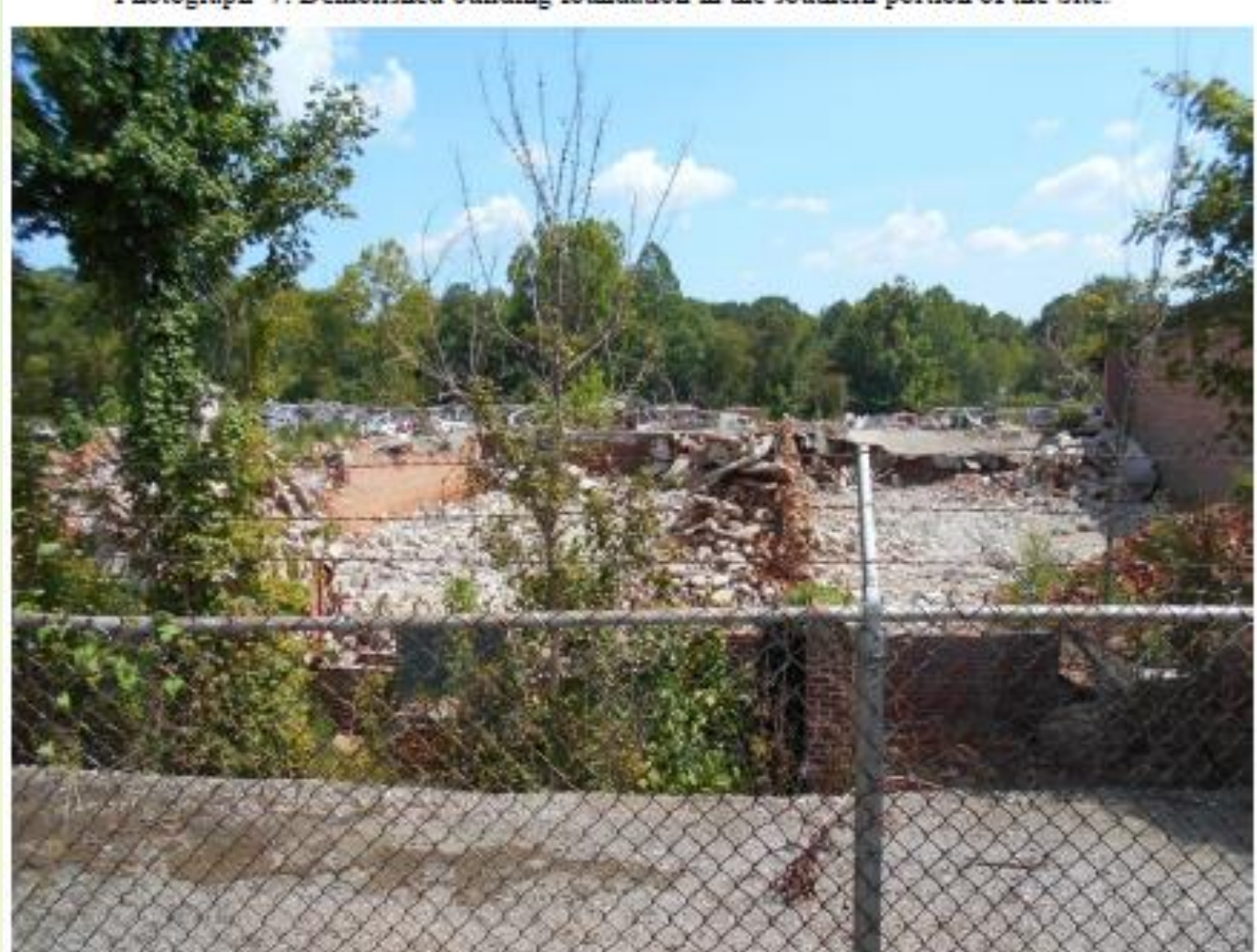
Photograph 8: Demolished building foundation in the central portion of the Site.
