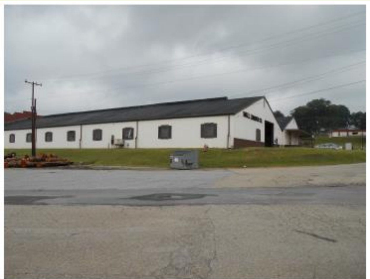
Photograph 11: Wall Lumber Company to the north.
