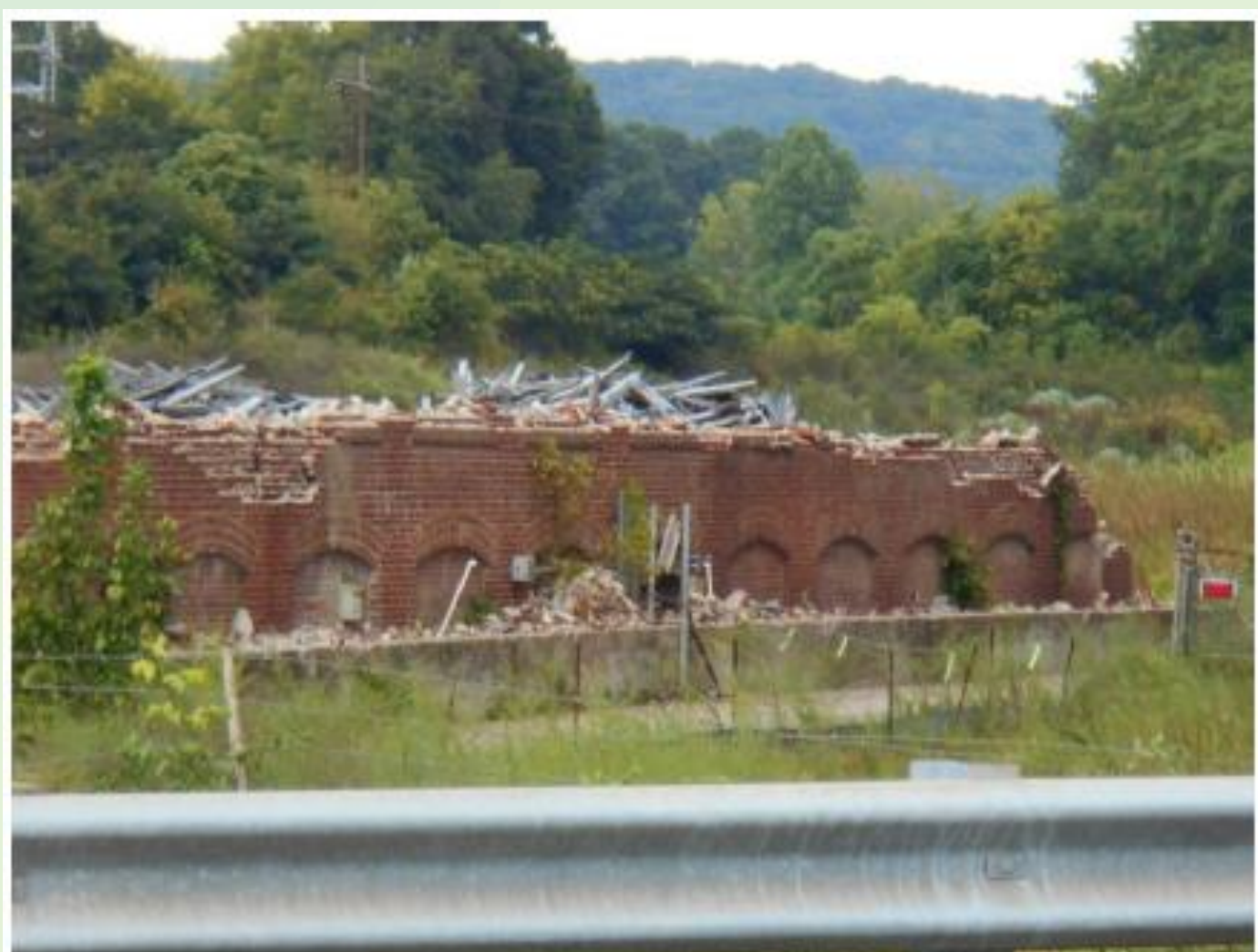
Photograph 7: Demolished building foundation in the southern portion of the Site.
