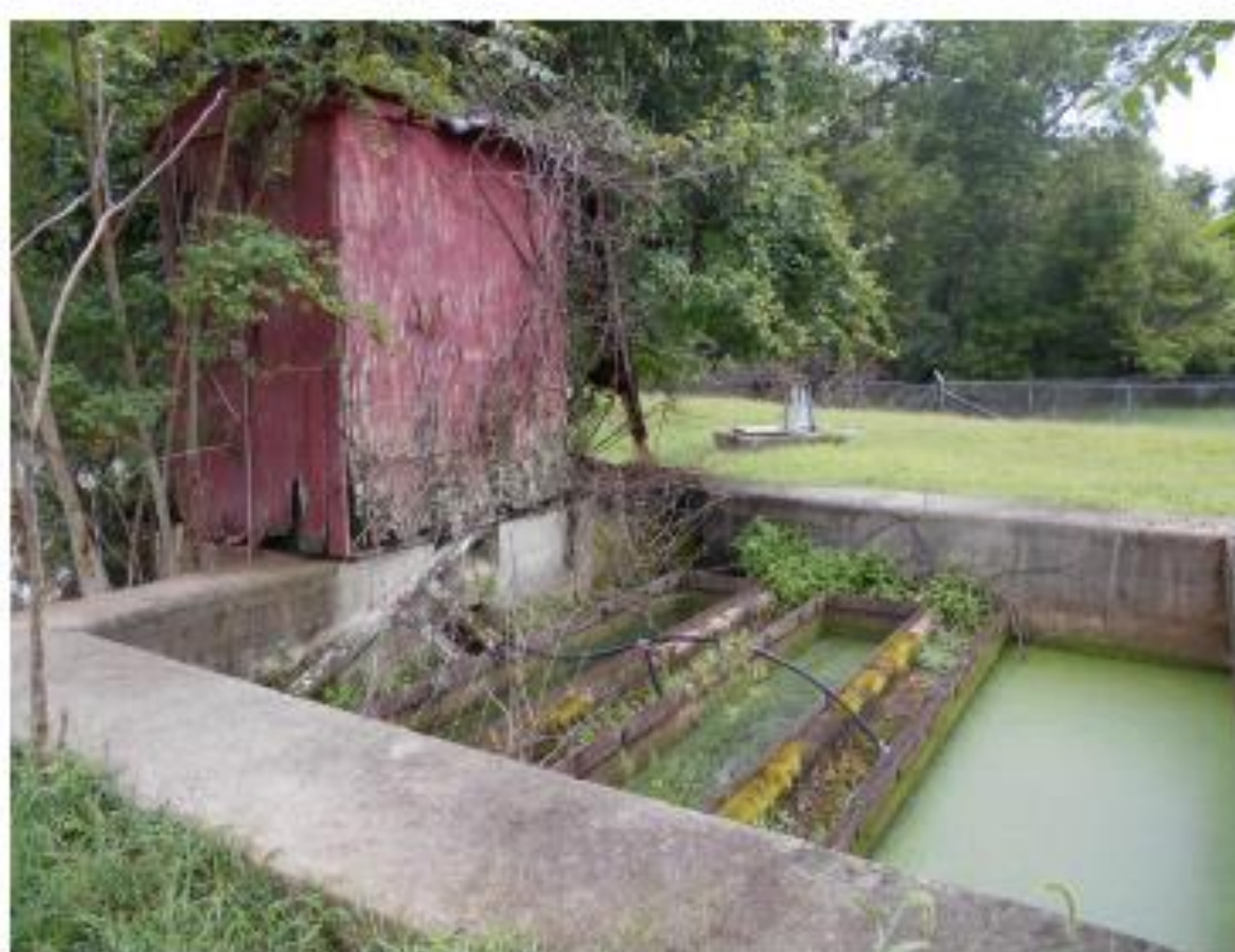
Photograph 4: Chlorine gas storage building.
