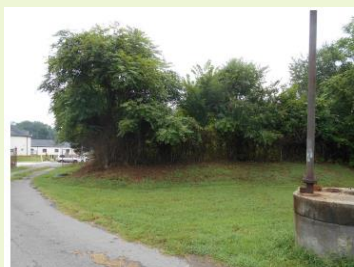
Photograph 5: Location of the concrete lined retention basin.
