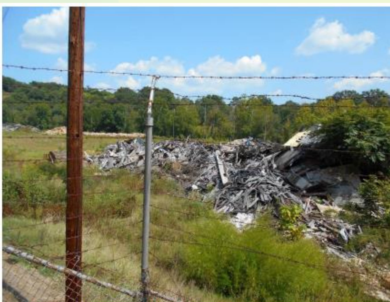
Photograph 9: Typical debris pile located in the southern and central portions of the Site.
