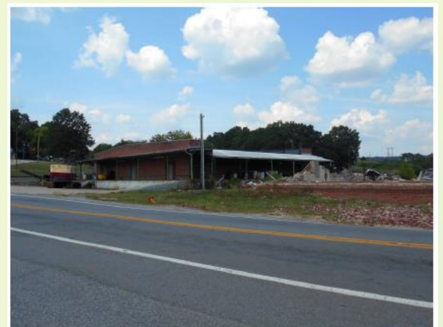
Photograph 5: Remaining Site building in the southeastern portion of the Site.
