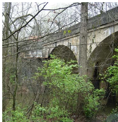
Railroad Bridge over the Deep River
