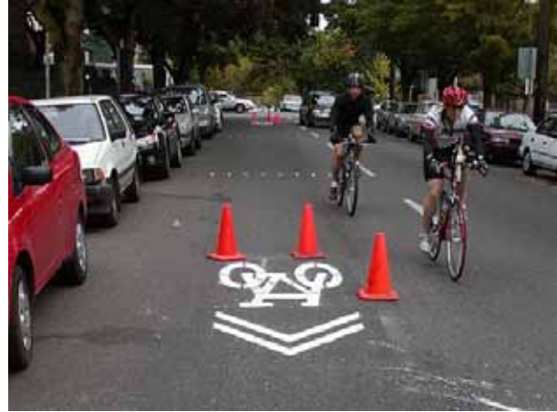
New sharrows in northwest Portland, OR (Source: www.bikeportland.org)
