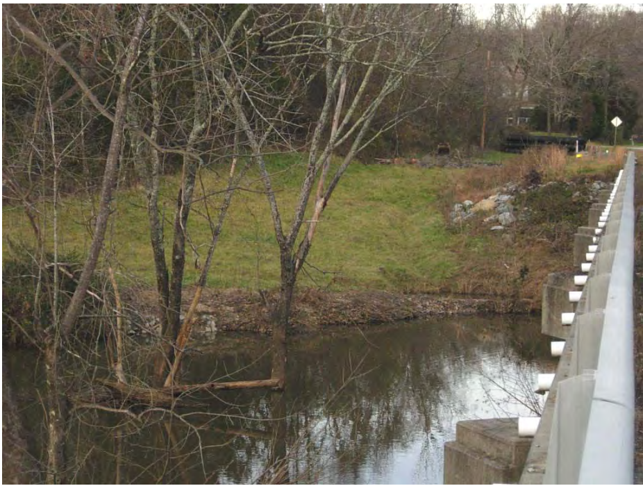
3. Potential River Access Looking East at Kivett Drive
