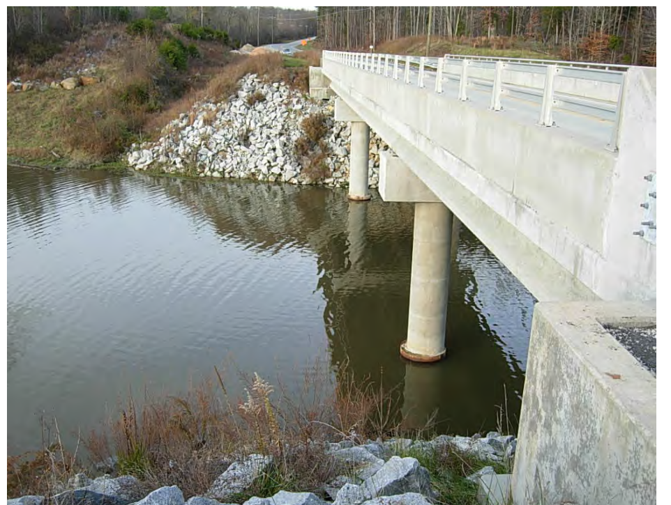
6. Groometown Road Bridge Over Randleman Lake Looking East
