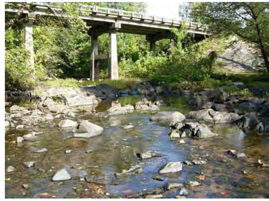
14. Deep River south of Harvey Road bridge, shown here in Fall
