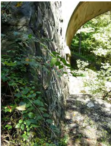
5. Area under NC Railroad bridge looking north
