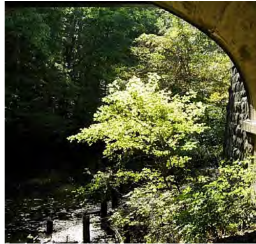
4. Area under NC Railroad bridge needing improvement looking south
